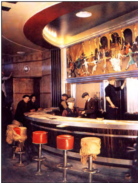
The Queen Mary Round Bar with installers and workmen, 1936.
