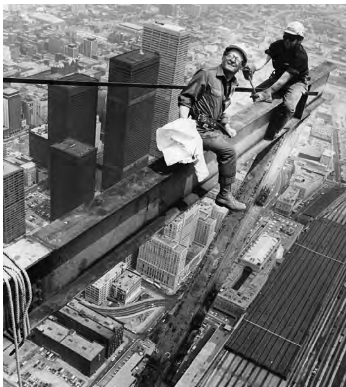
Construction of SkyPod by Boris Spremo, 1974.
